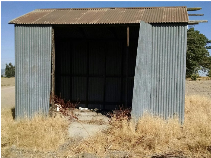
Shed near barn, camera facing north (SWCA photo, 9/19/2018).
