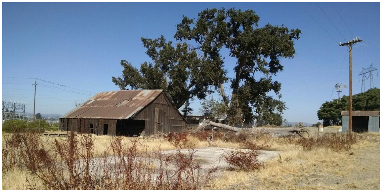
Figure 6. View of barn located at 1210 El Pomar Drive
